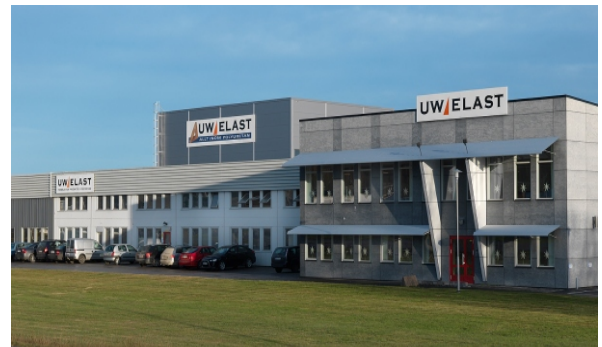
UW ELAST's factory in Mariestad is the largest unit of solid cast contract production in Sweden.
